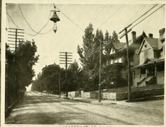
JEFFERSON ST. VIEW
